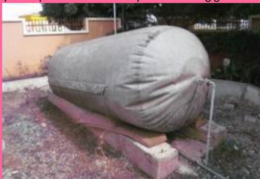
Biogas storage balloon in the corner of the car park of the African Regent Hotel
