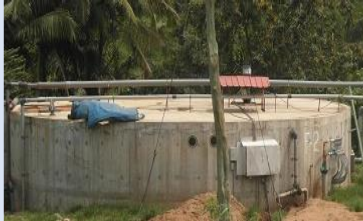
Stirred-tank digester, HPW Fresh & Dry Ltd., Adeiso, Ghana
